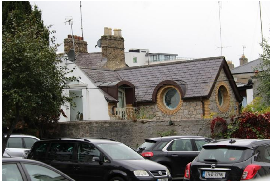
Plate 10: Rear of mews terrace, seen from application site
