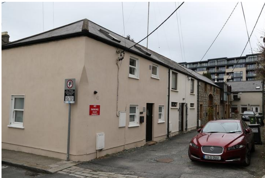
Plate 8: Mews at rear of Charlemont Terrace
