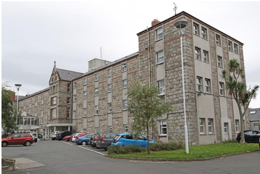
Plate 4: Hospital building to south of application site
