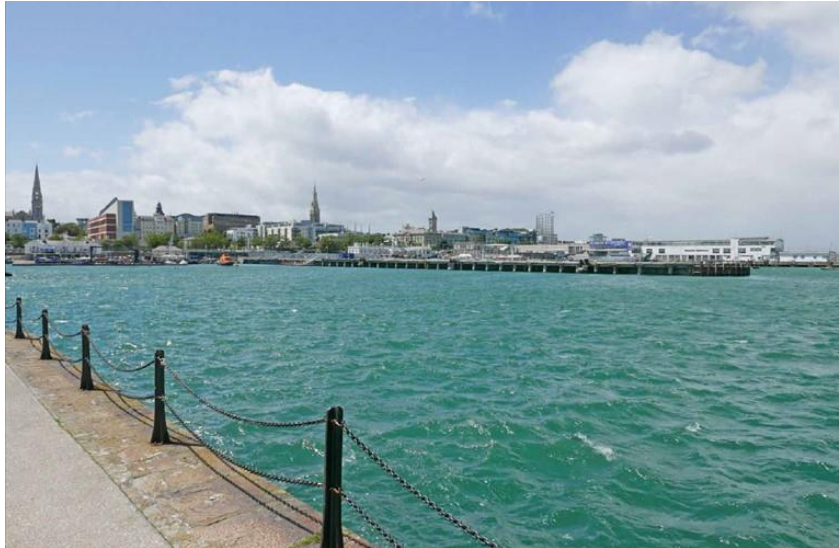
Plate 18: View 11, from the East Pier with the proposed building at right
